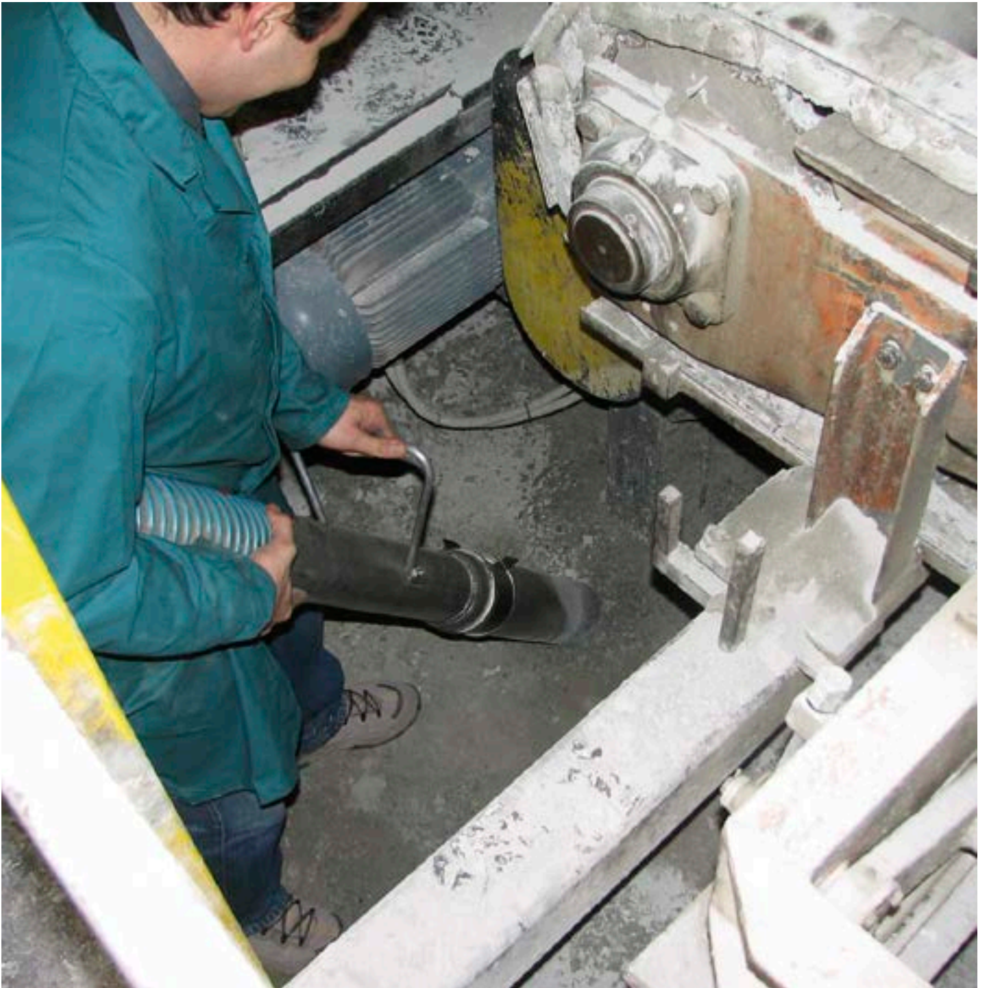
Cement: trench cleaning.
